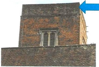
Crumbling tower bricks & mortar
