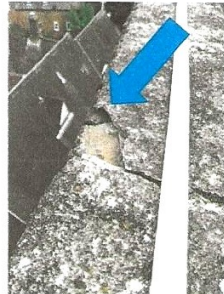
Broken parapet
