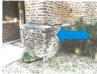
Broken parapet
