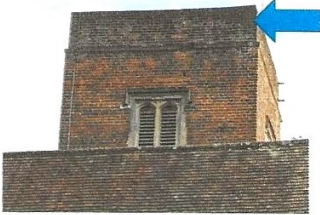
Crumbling tower bricks & mortar
